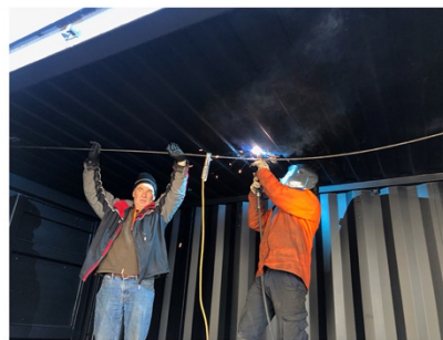
Curtain rail under construction.
